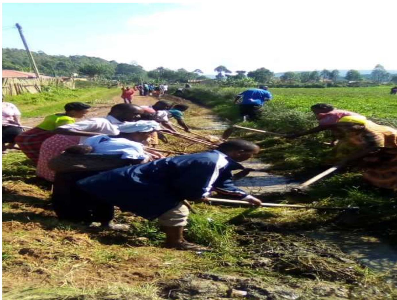
Figure 2: Community members making water trapping trenches.
